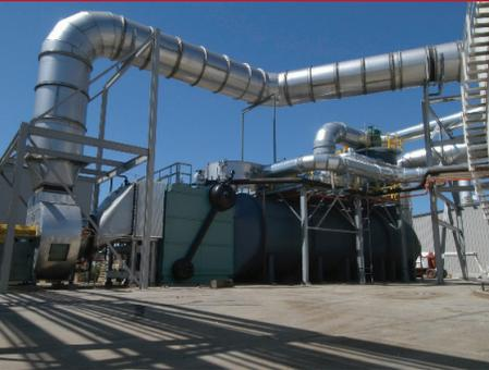
The steam generated from this recovery is applied to the fermentation, refining and drying processes that convert the liquid-laden corn byproduct into dry cattle feed that can be easily stored and shipped.
